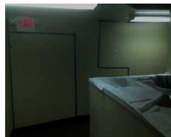
Taped wall to mark construction for HCHC's dental wing.
